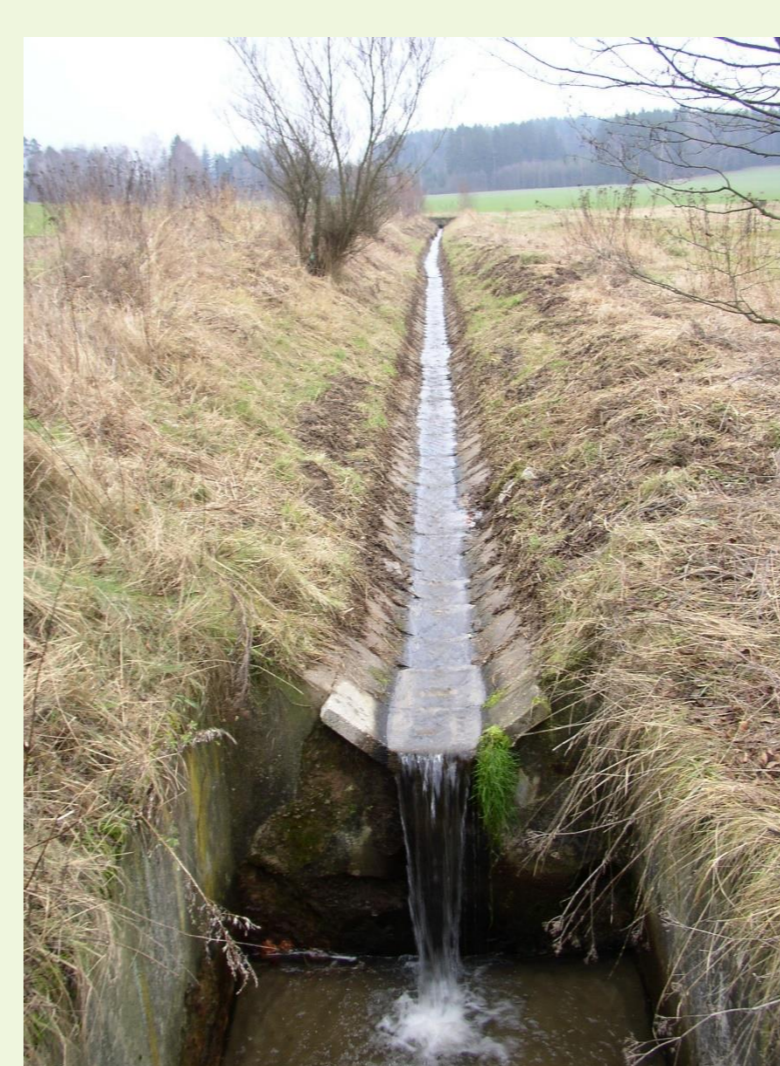
◀ Straightened and deepened small waterways
